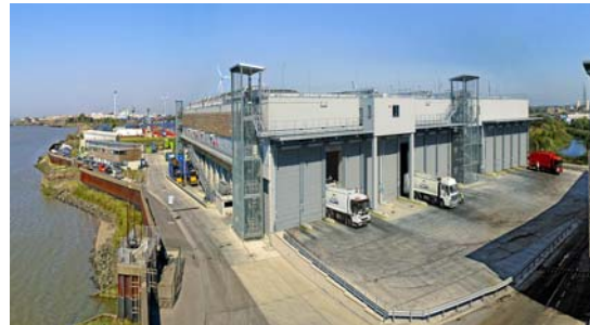
Frog Island Waste Management Facility
